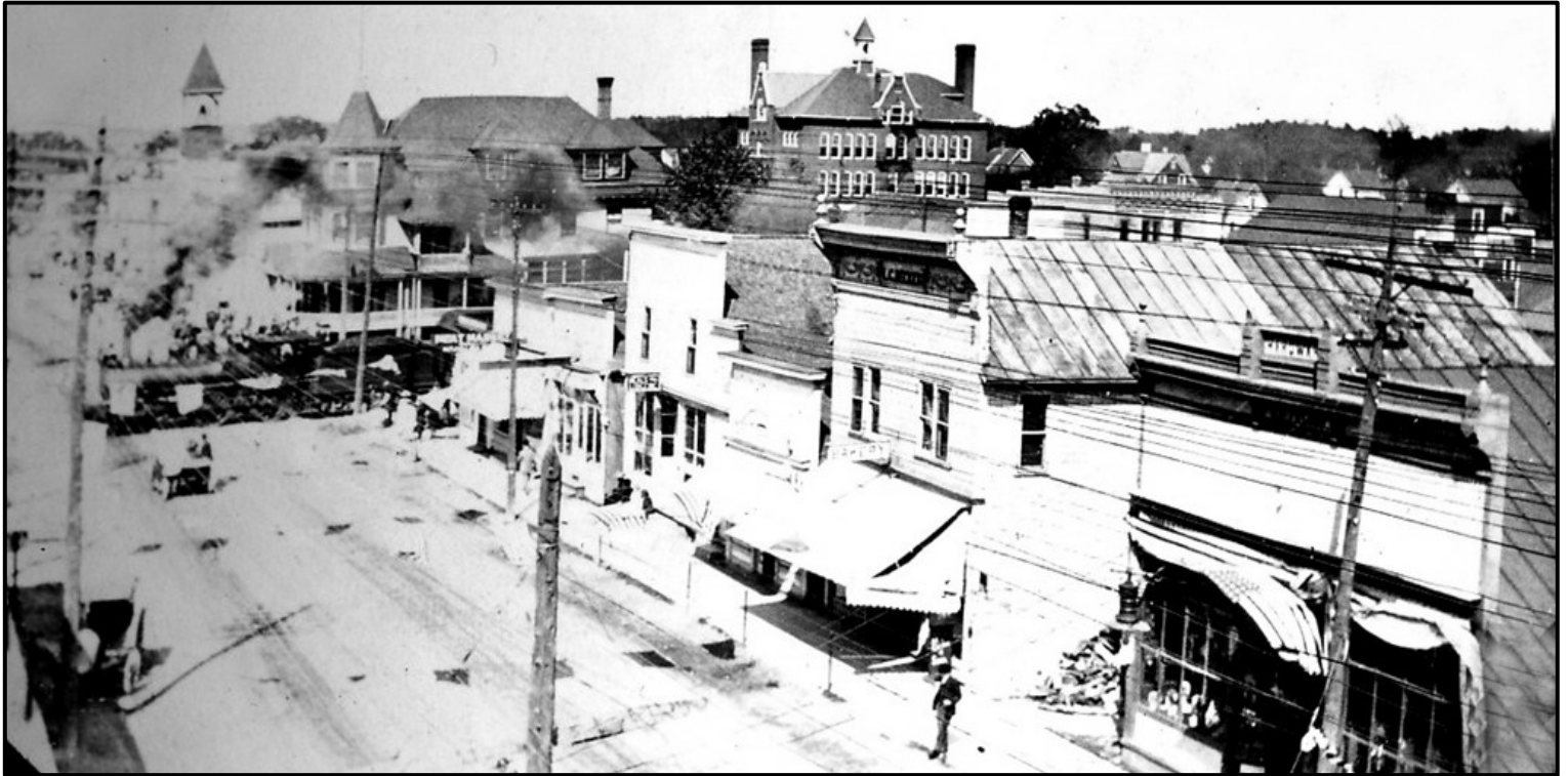
This view looking north on Main Street shows the smoke generated by the locomotive as it pulled away from the depot. Notice how the school, city hall, and Seymour Hotel dominated the landscape. Businesses visible on the east side of Main Street include Feurig Hardware, Becker's Home Bakery and Hallada's Meat Market.
