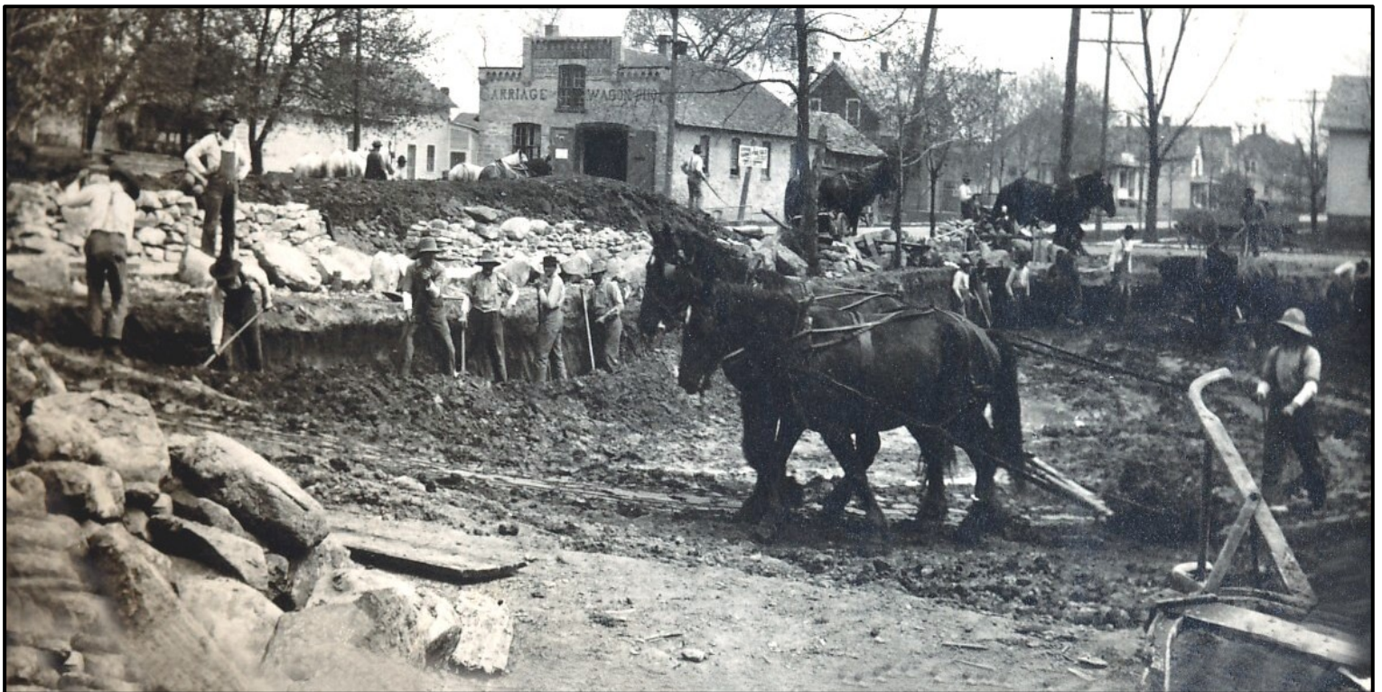
This is a picture of the excavation of the foundation for the Emmanuel Lutheran Church on northwest Main Street. It clearly indicates how horses were used to pull a large bucket that removed the earth. Notice the men with shovels getting ready to take on the backbreaking work.
